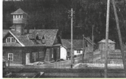
Ostrelj with electric street lights from the Austro-Hungarian era
